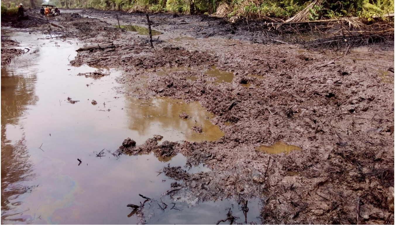
Fig E: Backfill after repair of incident facility
