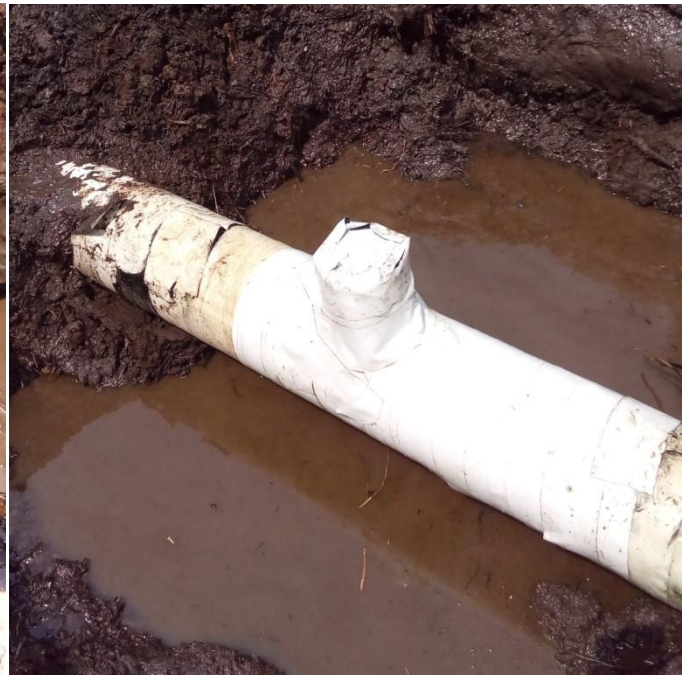
Fig D: The Spill Point after repair
